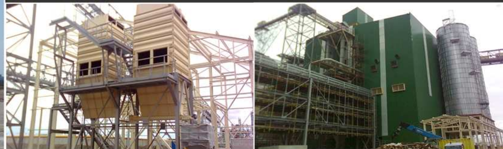
ROTTERDAM, PLANTA BIODIESEL, 2009.
